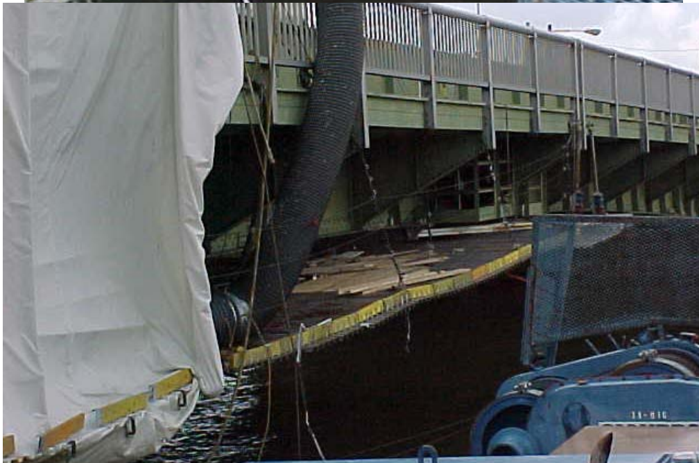
SOUTH MARKET STREET BASCULE BRIDGE New Castle County, Delaware
